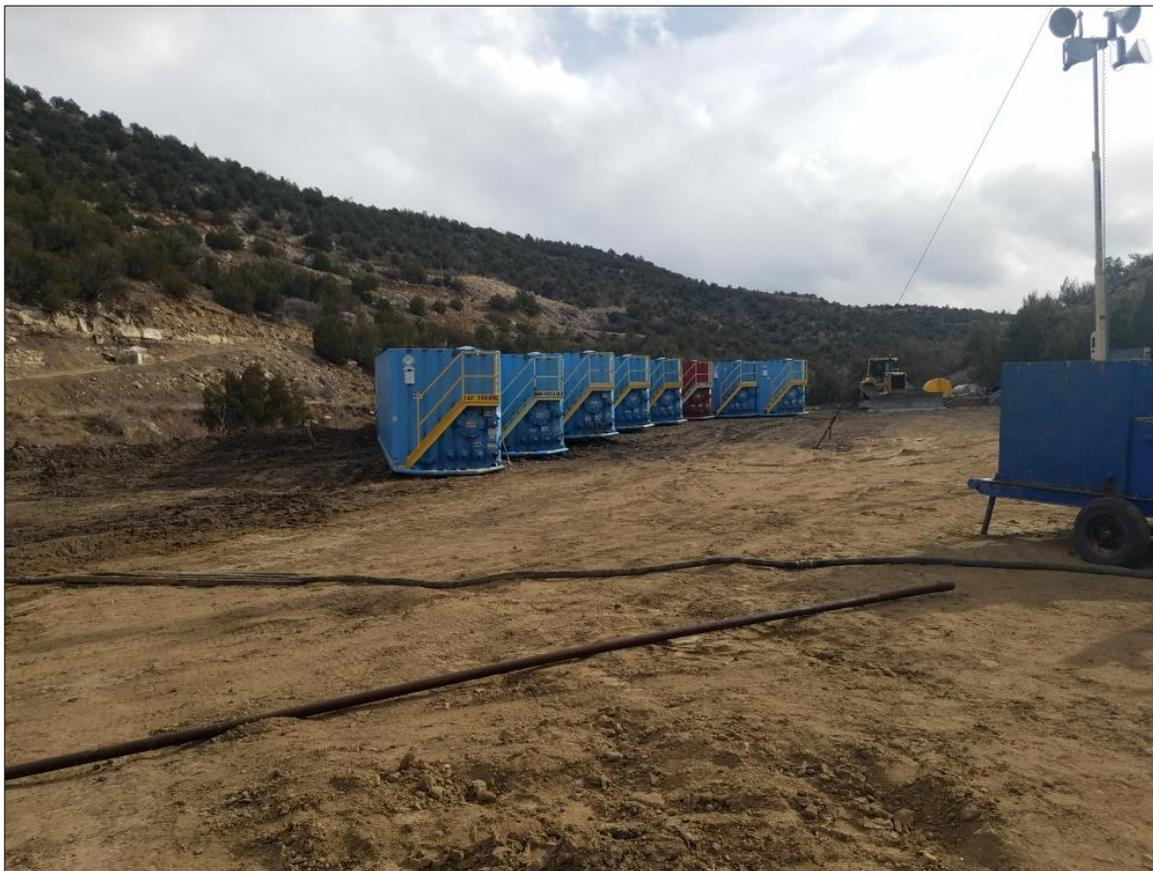
**Figure 2:** Several frac tanks in place for fracture stimulation operations.
